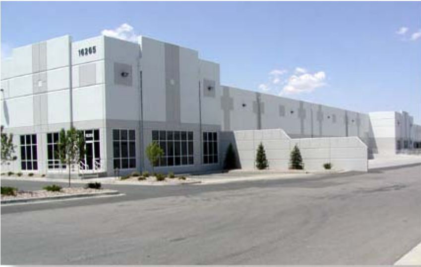
Gateway Park Building 15
